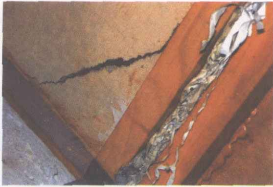
图 4 壁画接缝内充填的纸屑 Fig.4 Wastepaper in joint of wall paintings
