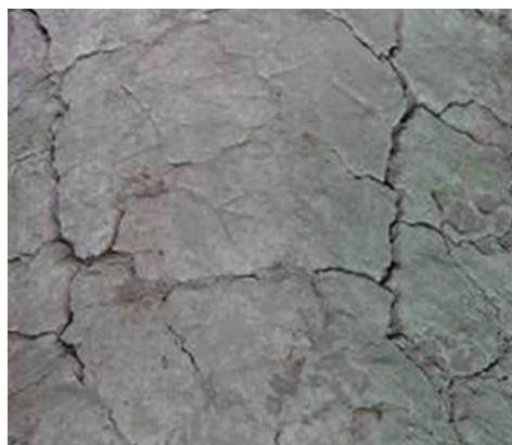
图7 壕沟边缘土壤裂缝 Fig.7 Ditch edge soil crack
