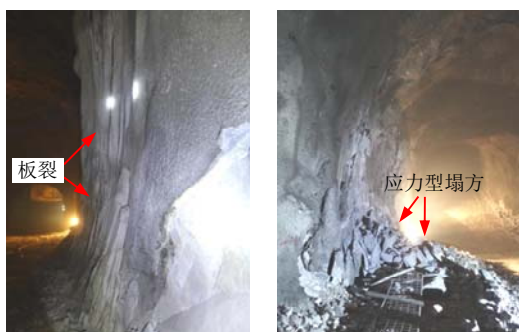
图 22 中国锦屏深地实验室开挖过程中围岩破坏现象 Fig.22 Failure phenomenon of surrounding rock at Chinese Jinping underground deep laboratory
