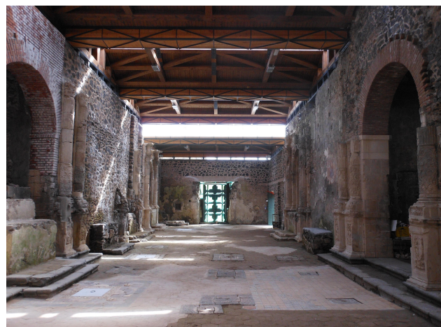
Figure 5. Interior of the church
