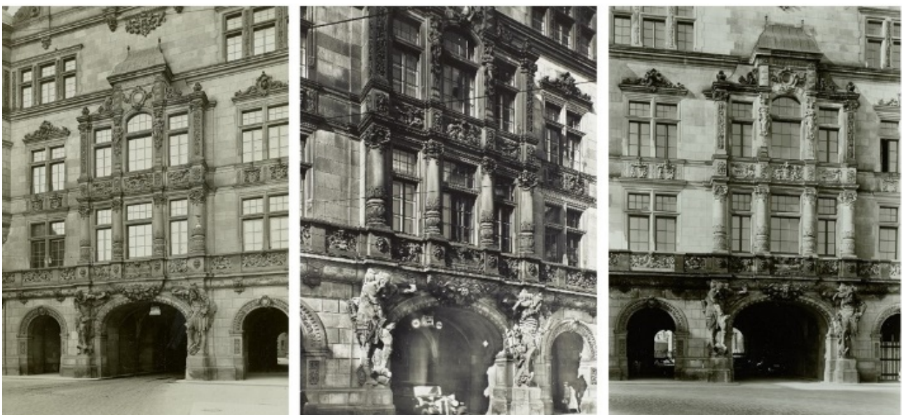
Figure 1. Example that shows radiometric differences between three historical images of the same building
