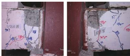
Fig. 15 Joint damage under 1/25 loading drift ratio
