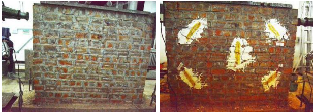
图 8 4-M4-RRBB2 墙体破坏照 Fig.8 4-M4 wall damage photos
