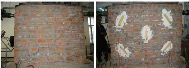
图 16 8-C1 墙体破坏照 Fig.16 8-C1 wall damage photos
