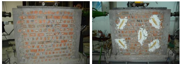
图 24 12-C5-RBCC2 墙体破坏照 Fig.24 12-C5-RBCC2 wall damage photos
