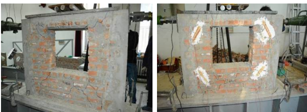
图 22 11-C4-RBCC1 墙体破坏照 Fig.22 11-C4-RBCC1 wall damage photos
