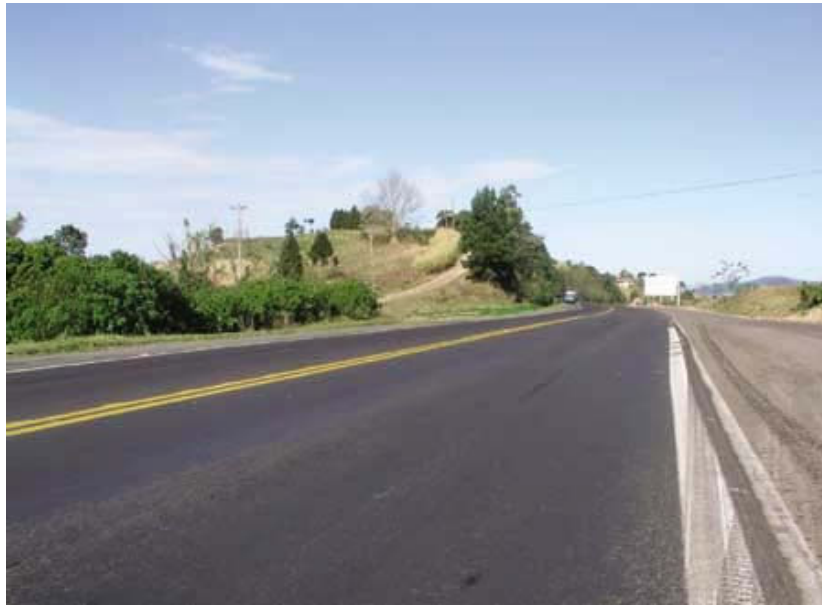
Figure 4 - Road with asphalt made with tire rubber
