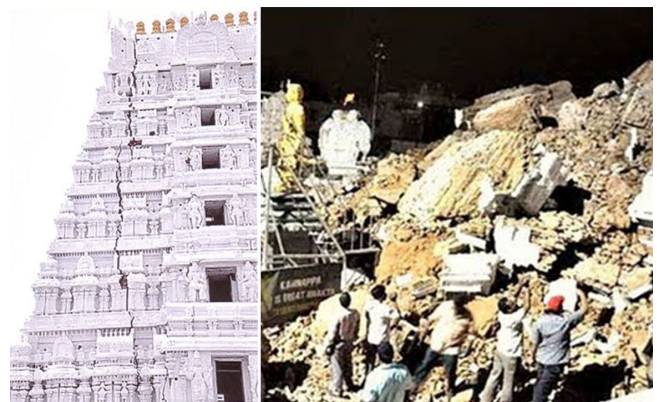
Figure 3 Gopuram before and after collapse (V.Sundaram, 2010)
