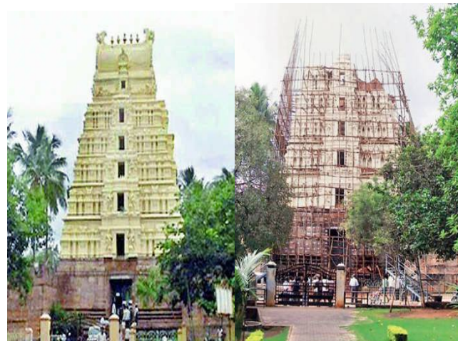
Figure 5 Shivaji gopuram – before and after collapse (indiatemplesinfo, 2012)
