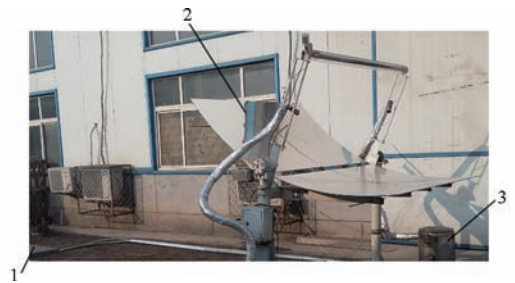
Fig. 11 Photo of PTC heating anaerobic reactor
