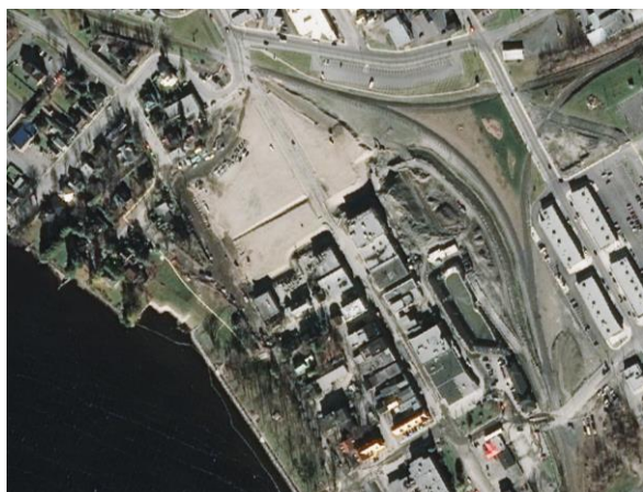
Figure 20. This Pléiades image Acquired on November 3, 2014 illustrates the progress of the remediation 16 months post-derailment. © CNES 2014, Distribution Airbus DS
