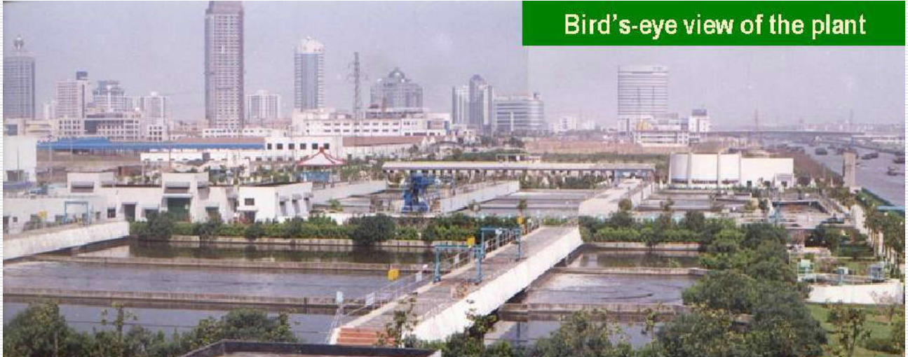
SND WWTP(three-alternate-oxidation ditch process), Suzhou, Jiangsu, CHINA
