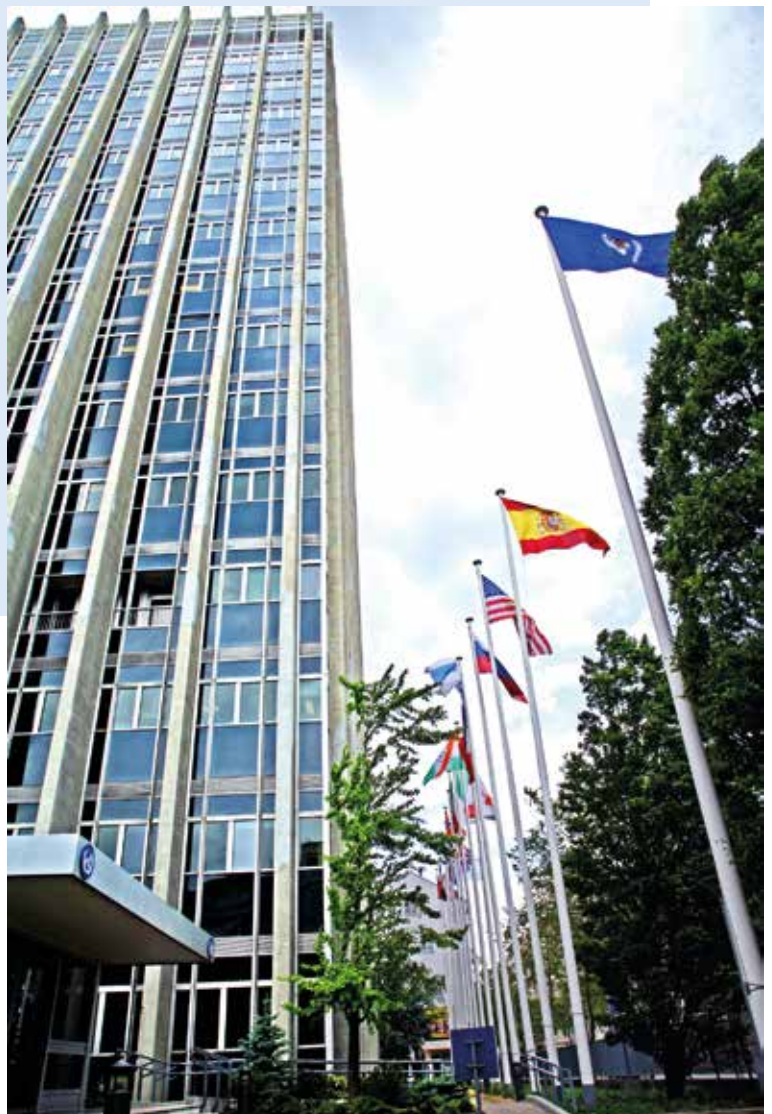
The IARC tower building in the eighth district of Lyon, with the waving flags of the World Health Organization and of the 24 IARC Participating States.
