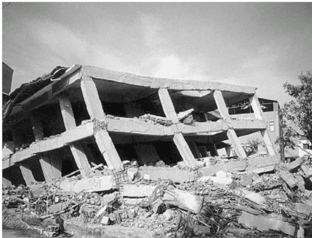
Fig. 1. Exterior joint failure during the 1999 Kocaeli (Turkey) earthquake.
