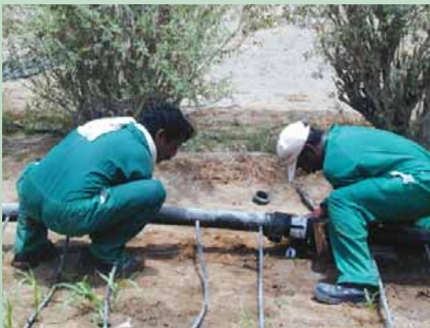
Installing irrigation system at the Dibba fram
