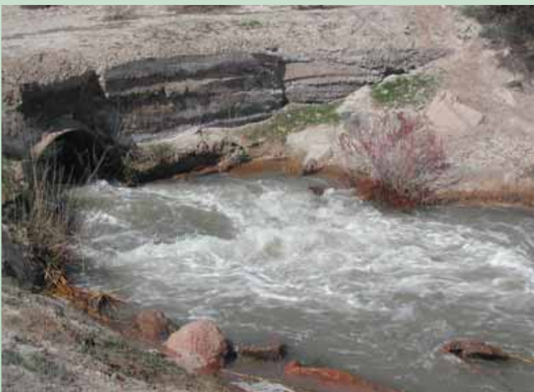
Drainage water from agricultural farms with low to moderate salt content can be used for on-farm management in Khudjand district
