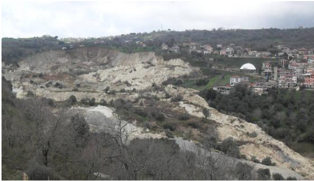
Figure 2. Panoramic view of the Maierato Landslide
