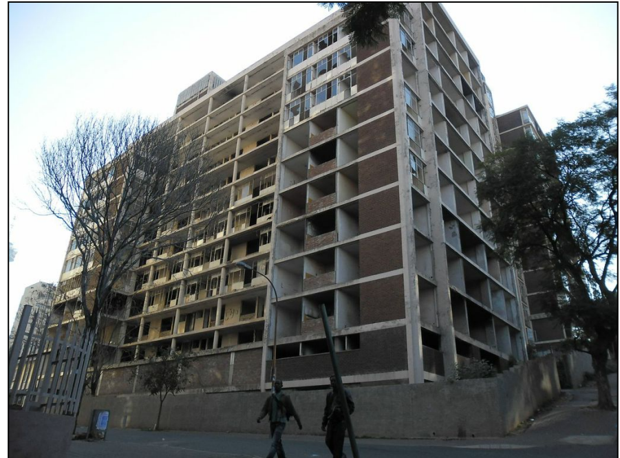
Figure 9 – San Jose Building, Berea, © Sack 2013.
