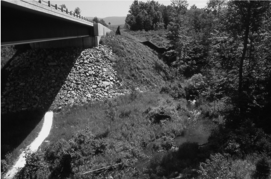
Figure 2.2. West Airport Brook (WAB) crossing structure showing rip rap slope, white track bed and perennial stream. Bennington, VT.
