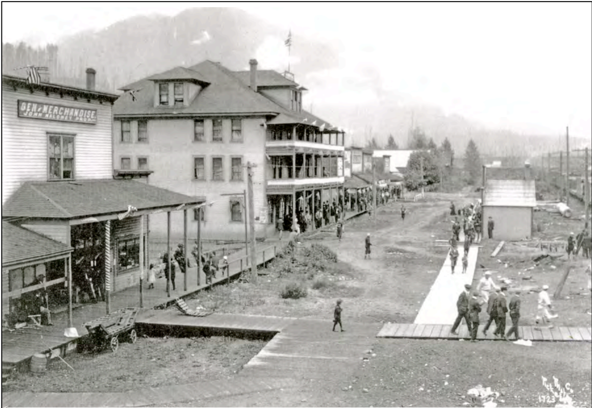
Figure 6. Skykomish, WA, c. 1913 , looking east with businesses on the left and railroad tracks on the right. Skykomish looks very similar today as it did in this historic photograph, but Maloney’s General Store (left) and the Skykomish Inn (center) are vacant. (Photographer, Lee Pickett; photo courtesy of the Skykomish Historical Society)
