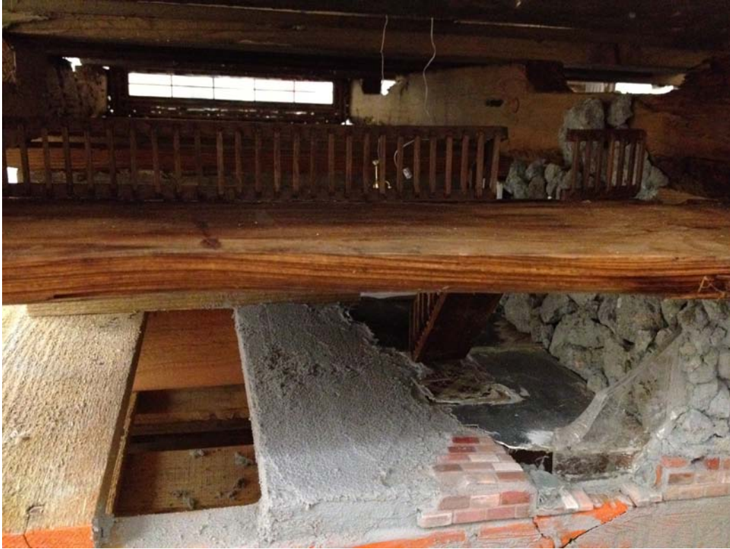
(Fig.31) Detail of Catwalk inside one of the pallet layers, 2012.
