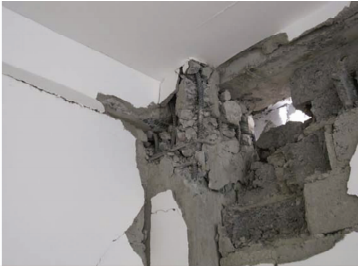
图1 框架柱头主筋压曲混凝土压碎 Fig.1 Concrete crushing and main bar buckling of column head in framework
