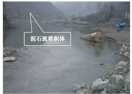
图10 蟹子沟泥石流形成堰塞湖全貌 Fig. 10 The full view of the barrier lake induced by the Crab Valley debris flow
