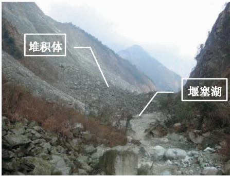
图8 堆积体堵塞黄梁沟 Fig. 8 Deposit blocks the Huangliang Valley
