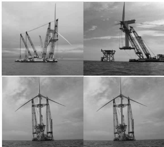
Fig.4 The overall hoisting process of Beatrice wind turbines
