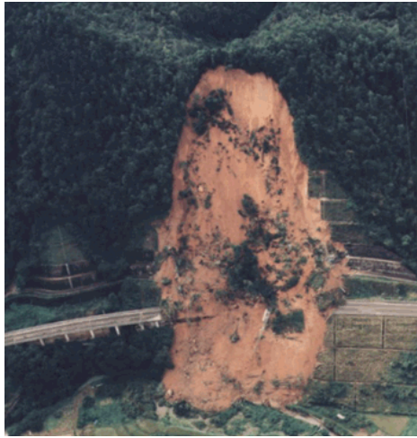
图3 斜面破坏后的情景 Fig.3 Scene of the slope after failure
