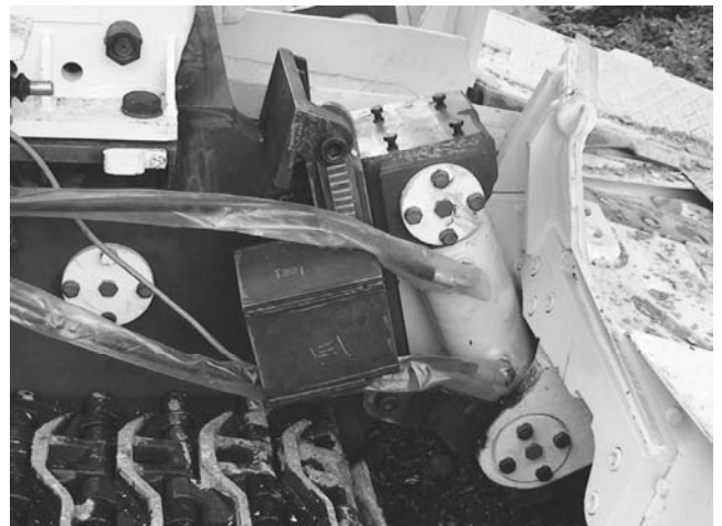
Fig. 11. Installation of loading table position sensor
