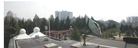
FIGURE 26: Environment at the Wuhan antenna site.
