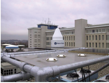
FIGURE 2: Space Engineering antenna mounted on the rooftop of the Septentrio office.
