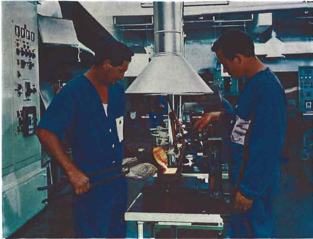
After chlorine refining, the gold, now of 99.6 per cent purity, is cast into 12.5 kg (400 ounce) bars. The furnace installation in the refinery consists of seven half-ton 150kW induction refining furnaces and two one-ton 225kW holding furnaces.
