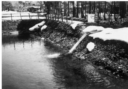
Photo 2-1 Basin No.2, the side of water supply, Apr. 5, 2001
