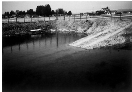
Photo 2-2 Basin No.2, the side of taking out sediment, Apr. 5, 2001
