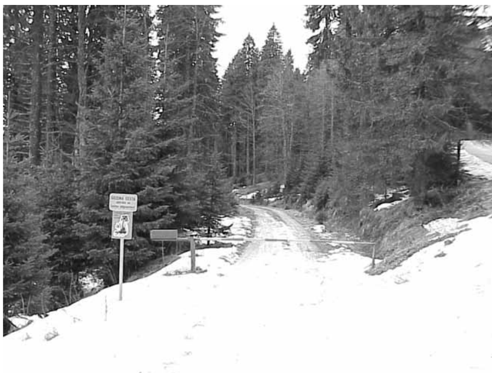
Fig. 3 Road barriers are an effective means of traffic regulation if implemented thoroughly
