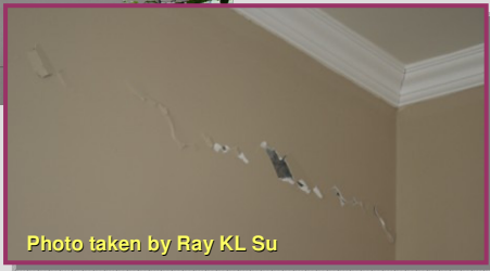
Damage at the interface between RC part and the brick work
