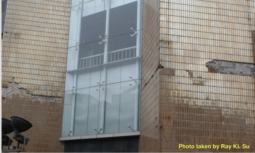
Tiles damaged but not glazing
