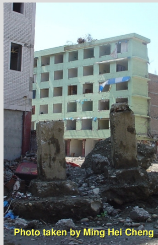
Typical column foundations
