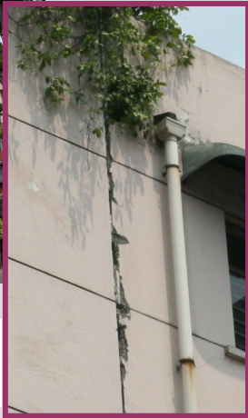
Pounding at the movement joint Damage to plaster
