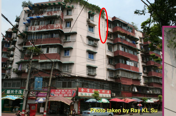
Pounding at the movement joint Damage to plaster
