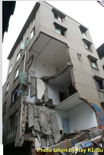
Partial collapse of a six storey building
