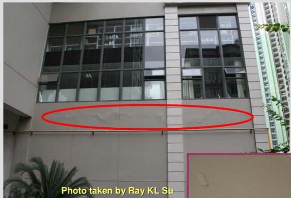
Damage at the interface between RC part and the brick work
