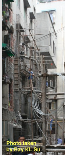
Strengthening of external walls and cantilevers
