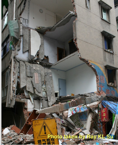
Partial collapse of a six storey building
