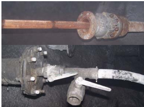
图 5 钻孔及注浆情况图 Fig.5 Drilling and grouting
