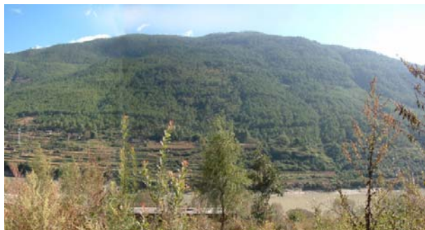
图 1 龙蟠右岸斜坡变形岩体全貌 Fig.1 Picture of the Longpan slope
