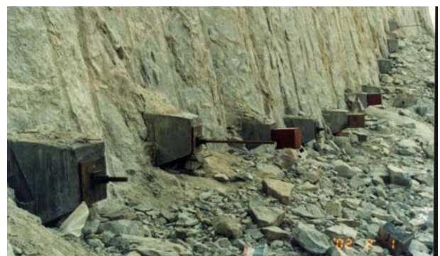
图 2 现场试验全貌 Fig.2 General view of in-situ experiment
