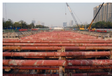
Figure 4. Site photo of steel supports 图 4. 现场钢支撑架设图
