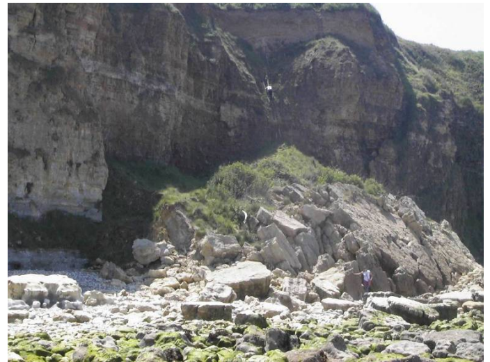
Figure 2: Massive collapse about 300m west of the O.P.
