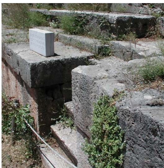
Figure 7. Formation of the retaining wall at Stadium in Delphoi
