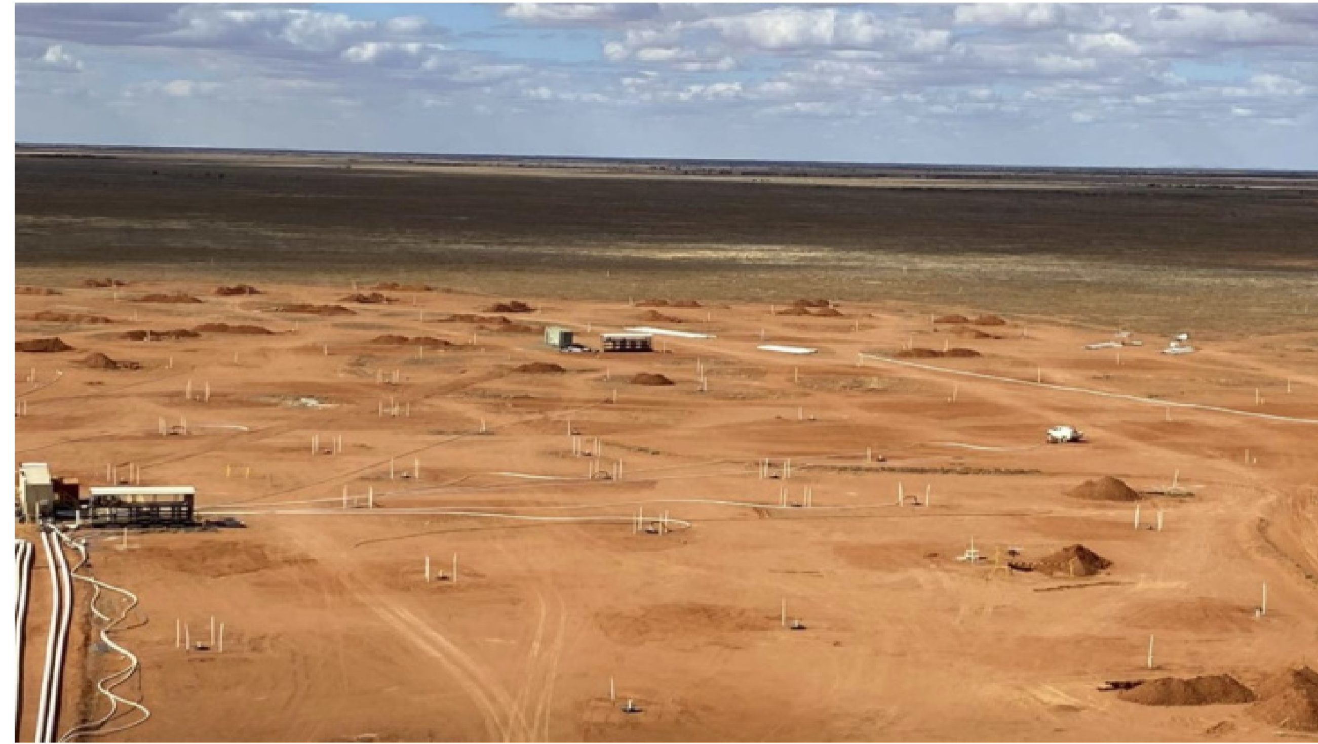
Construction of the three start-up wellfields at Honeymoon (Image: Boss Energy)
