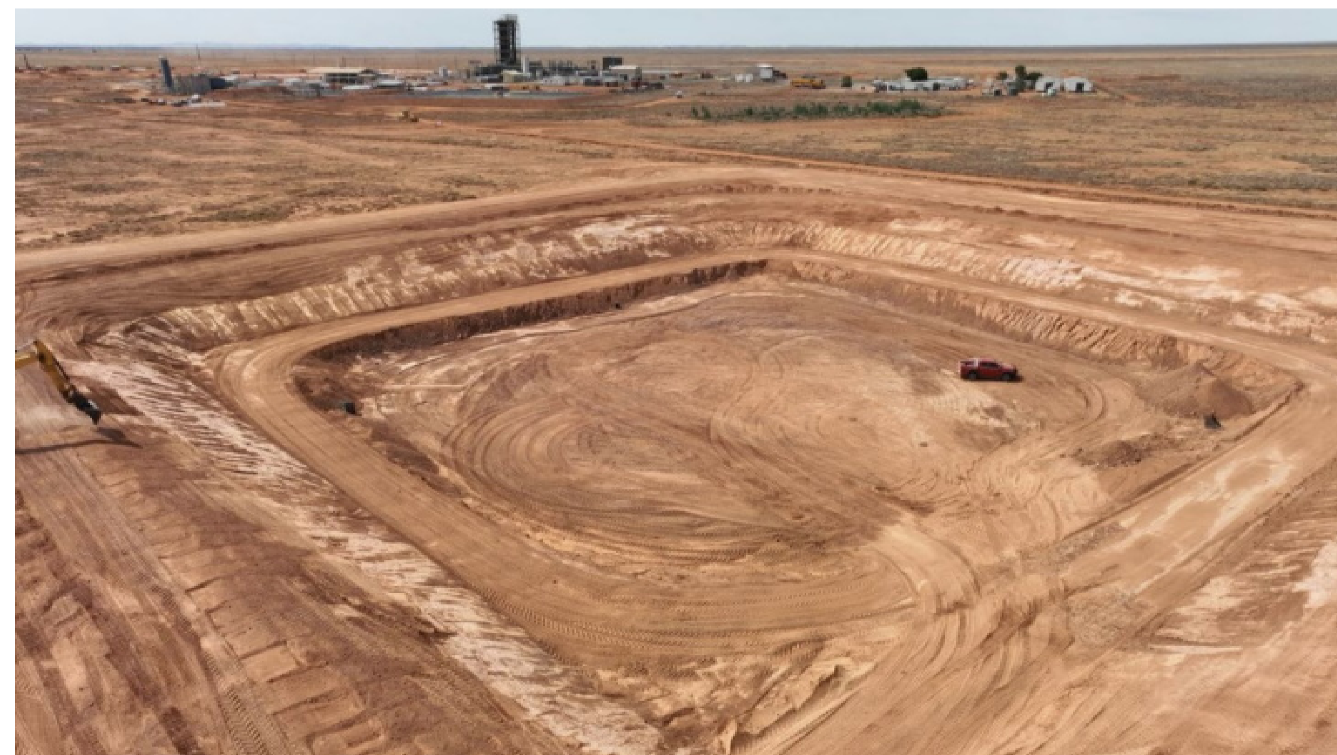
Excavation earthworks for the gypsum pond (Image: Boss Energy)
