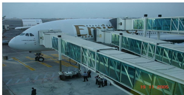
Figure 1. Combined aerobridge 图 1. 登机桥
