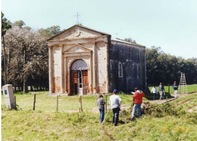
Figure 1. Saint Anthony's chapel façade
