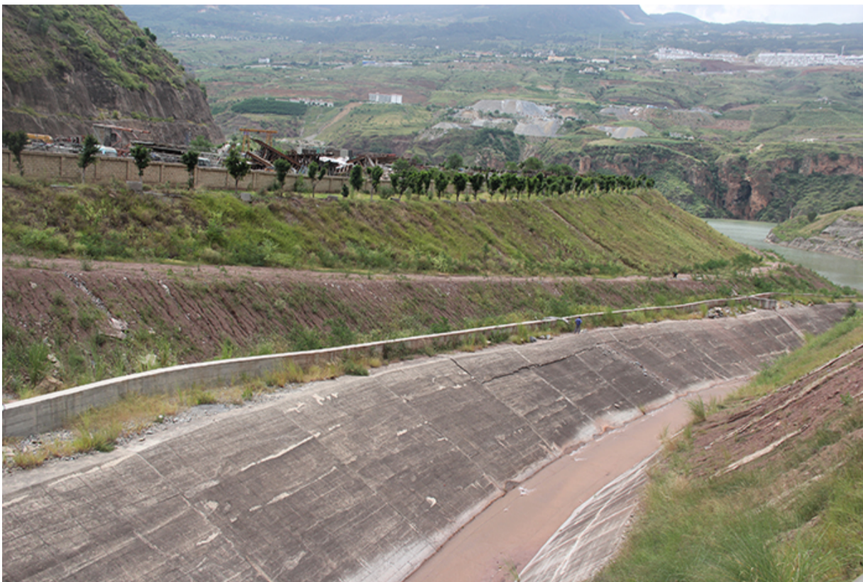
阴地沟弃渣场排导槽及边坡绿化
