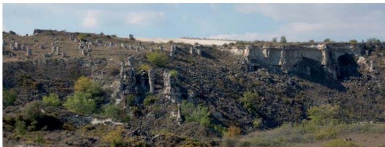
Figure 2. Overview of part of the Beloslav quarry from distance. The wall is approximately 35 m high. (photograph by A. Foubert).
