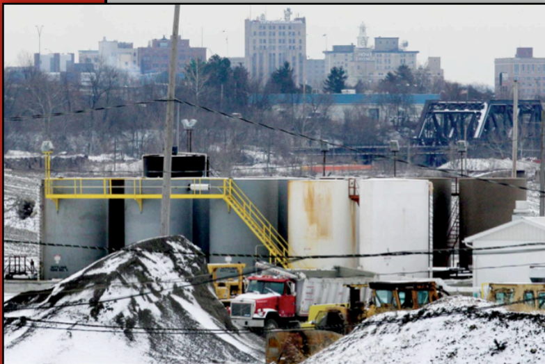
Left. A saline wastewater injection well owned by Northstar Disposal Services LLC in Youngstown, Ohio. Following several small earthquakes in the area in December 2011, the company halted injection of wastewater into the well, which stopped the earthquakes. The wastewater is from the production of oil and gas.
