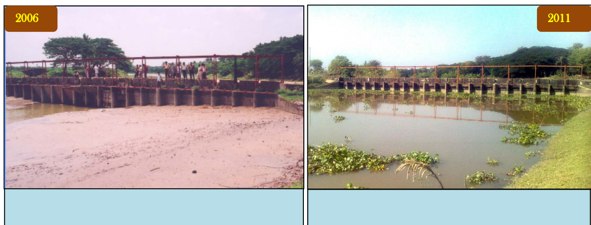
Figure 9 (a): Hari River near Babodaoh regulator before TRM Figure 9 (b) : Hari River near Babodaoh regulator after TRM
