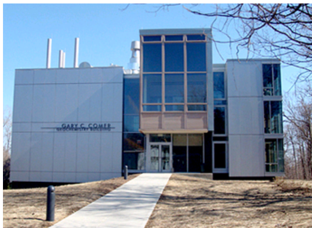
The 63,000-square-foot structure is designed for high energy efficiency and harmony with its rural landscape along the Hudson River
