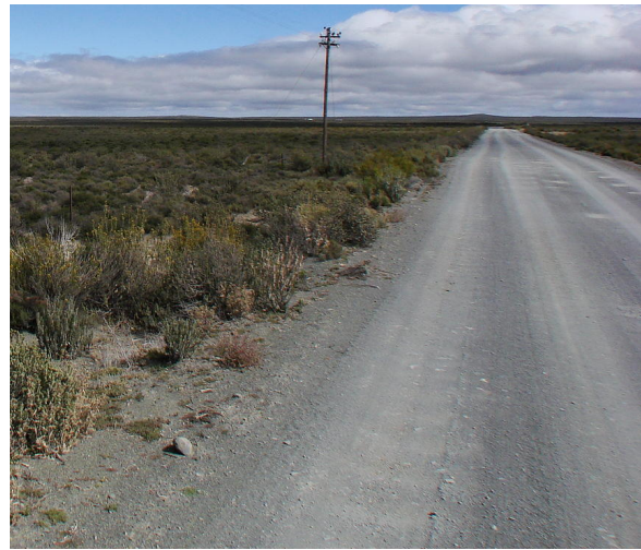
Figure 2.8: Gravel roads around Sutherland
