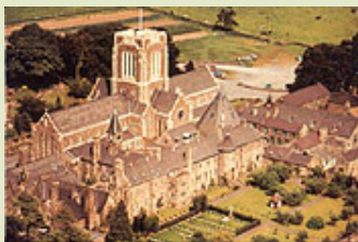
Fig. 8 The south front of Mount Saint Bernard Abbey, ca. 1990. Pugin completed the western portion of the church (left of the tower) and the cloister area attached to it. Between 1934 and 1939 architect Albert Herbert of Leicester added the transepts, tower, and eastern nave. Pugin's son, Edward Welby Pugin, completed the octagonal chapter house south of the tower transept in 1860. (Courtesy of the monks of Mount Saint Bernard Abbey)
